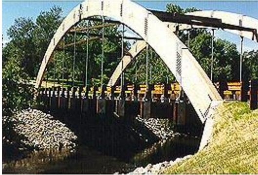
The Fontana Park Bridge is one of 419 demonstration timber bridges built since 1988. It has a record-long span for a bridge built with wood.
